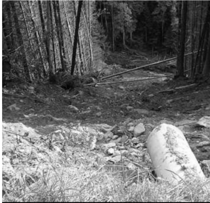
Fig. 7 – Landslide triggered off by improper forest road dewatering (Haslau 2005).
