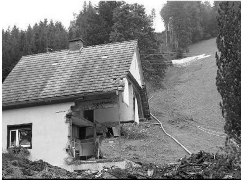
Fig. 1- Building badly affected by a landslide developing into a debris flow (Gasen, 2005). No information was available on landslide hazards in this area (neither any documentation from previous events nor from hazard mapping) although it is very likely (according to oral information and geomorphologic conditions), that landslide events had existed before.
