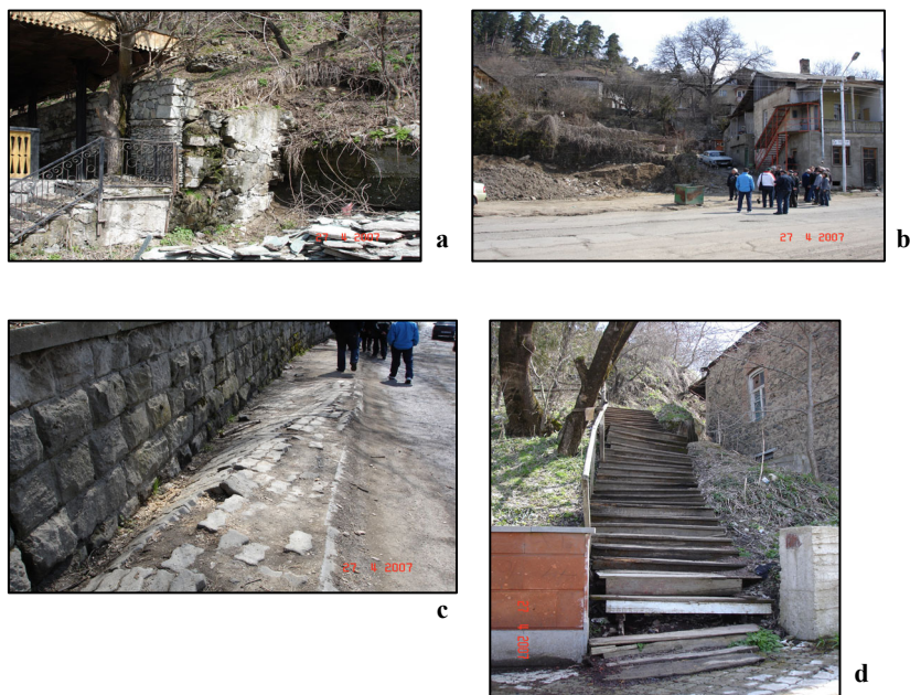
Fig. 11 – The consequences of displaced landslide masses in the town of Dilijan: a, b , landslide masses fall on streets and buildings; c , strained cover of street; d , strained stone stairs.
