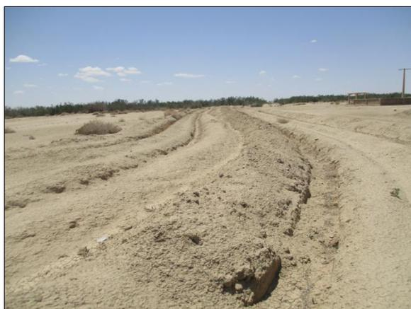
Fig. 8 – Floodwater diversion channels in the El Feidh perimeter.
